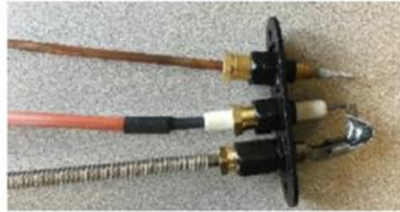
Pilot Mechanism Re-assembled
